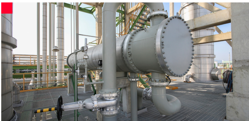
Figure 1. A typical heat exchanger. Undetected heat exchanger clogging hurts operational efficiency.
